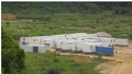
Turnkey Camp Project with Skids / Congo
