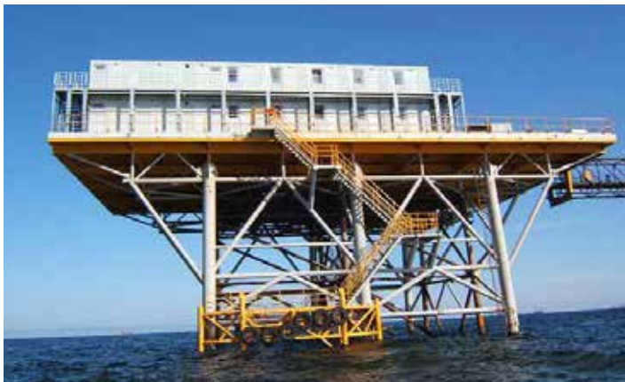
Offshore Container Camp / Turkmenistan
