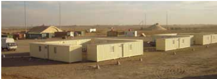
Accommodations modified from shipping containers
